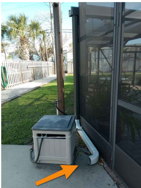
Gutter Downspout w/o Extension
