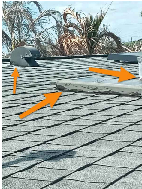
Skylight / Vent Flashing
