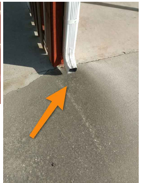
Gutter Downspout w/o Extension
