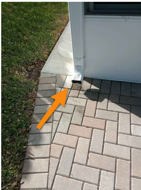
Gutter Downspout w/o Extension
