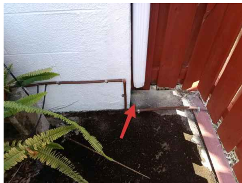
Gutter Downspout w/o Extension
