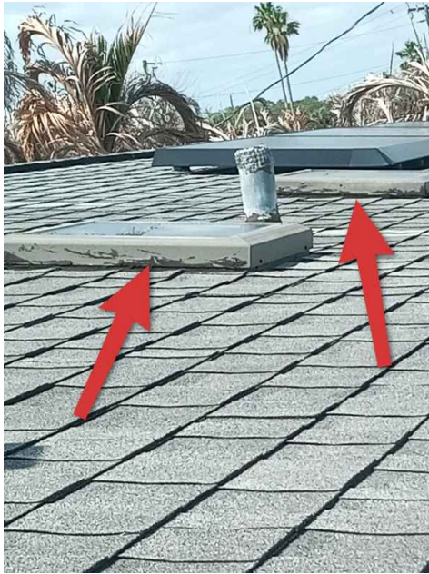
Skylight / Vent Flashing
